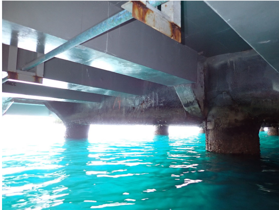
Photo 1: Typical Pier Substructure
